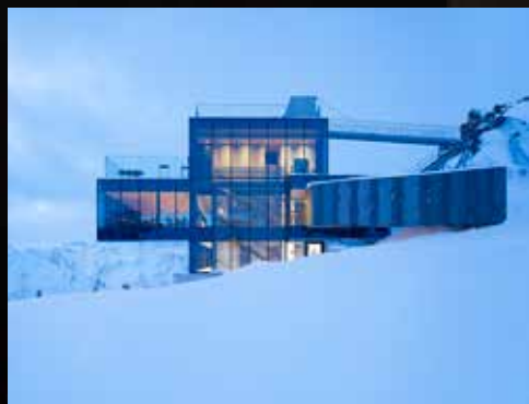
ICE Q SÖLDEN, AUSTRIA. ARCHITECT: JOHANN OBERMOSER
